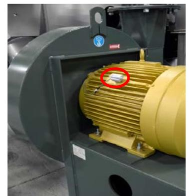
Fig. 1: Prophecy Sensor mounted on a blower
